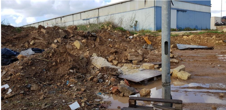
Figure 4: Photos of the Scheme site
