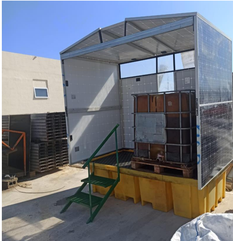
Figure 3.4: Waste oils storage
