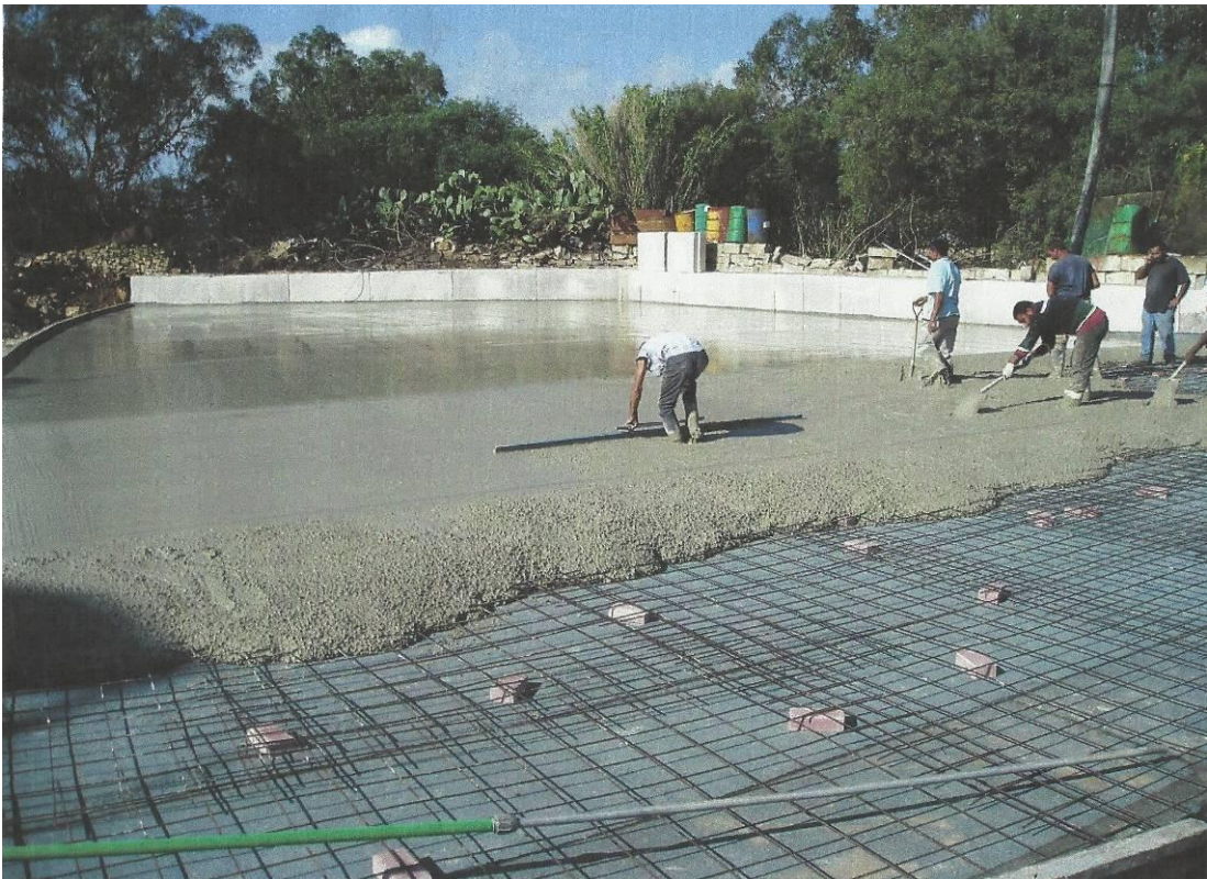
Figure 4.4: Installation of reinforced concrete surface
