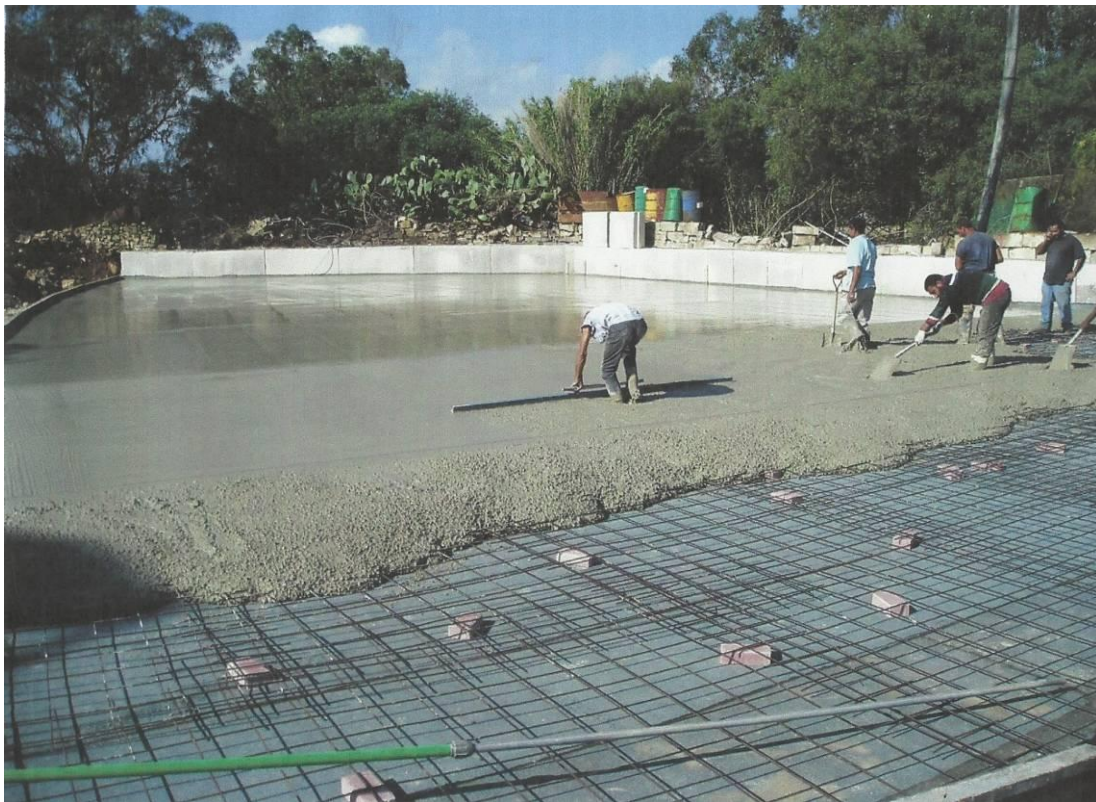
Figure 2.14: Installation of reinforced concrete surface
