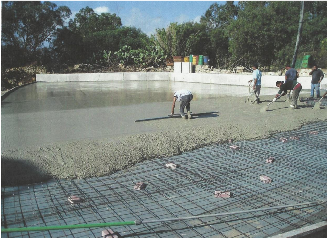
Figure 12: Installation of reinforced concrete surface
