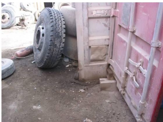
Figure 2.17: Oily stain near diesel tank
