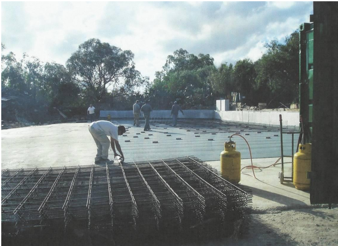
Figure 2.13: Installation of membrane underlay
