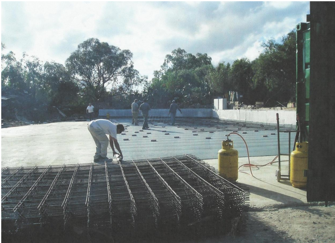
Figure 11: Installation of membrane underlay
