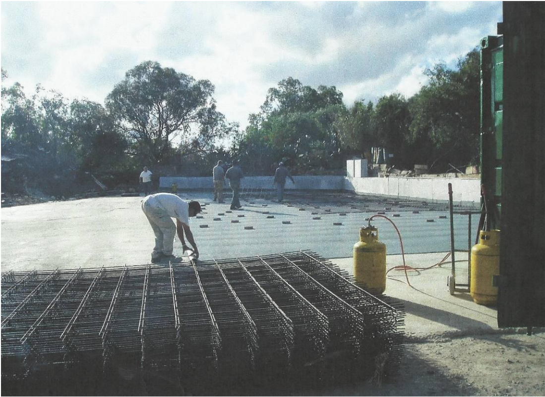
Figure 4.4: Installation of reinforced concrete surface
