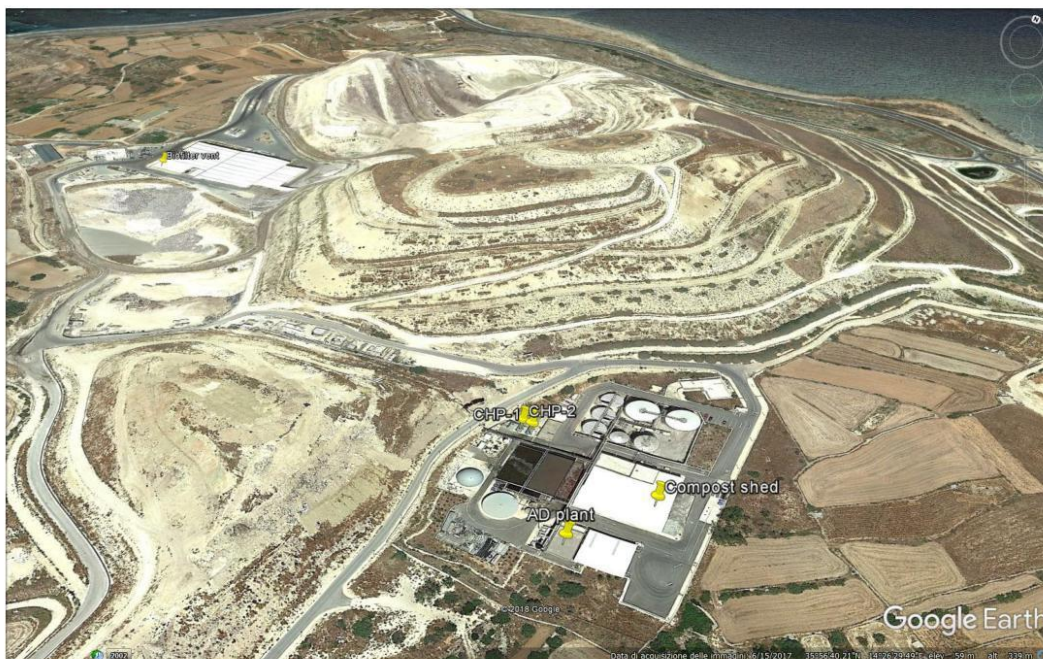
Figure 1: Malta North waste Treatment Plant
