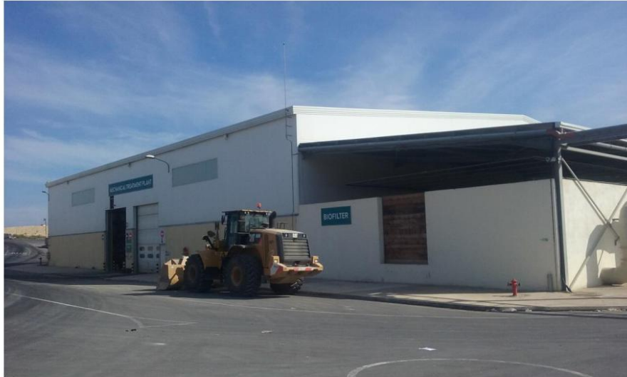
Figure 4: Biofilter vent (PS 7) sampling point
