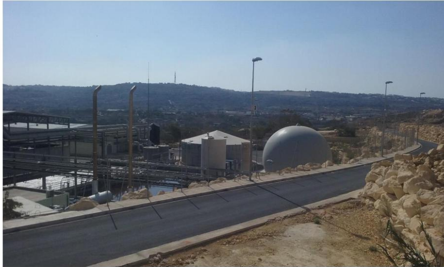
Figure 2: Stacks situated at the AD Malta North waste AD Treatment Plant
