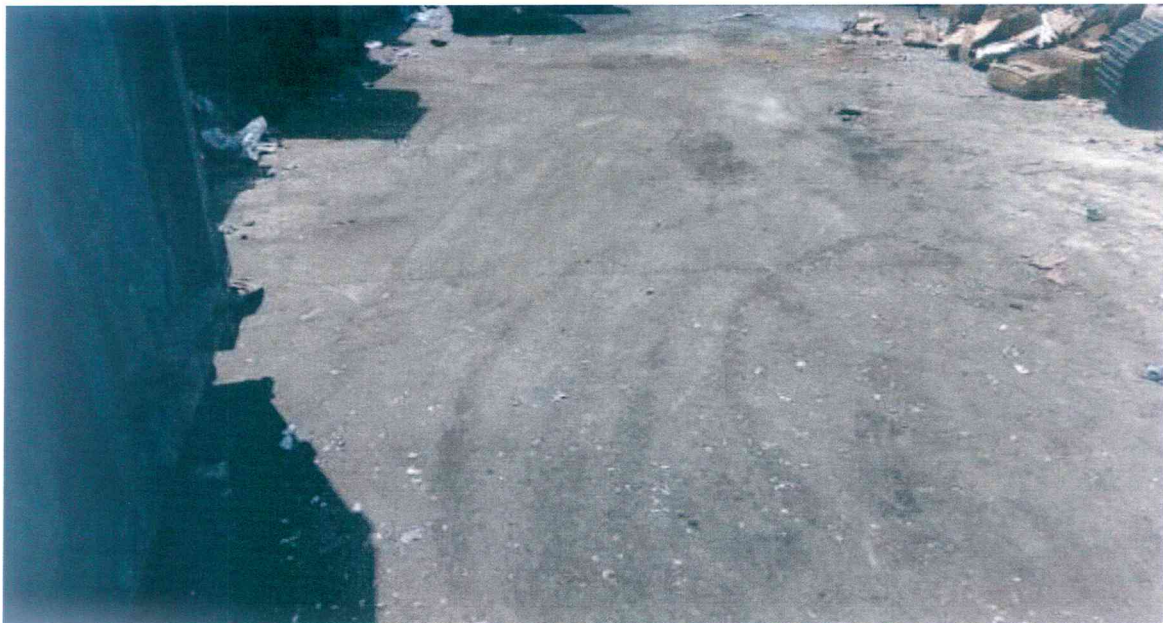
Figure 2: Location of separator 1 and discharge fluids pipework prior to excavation
