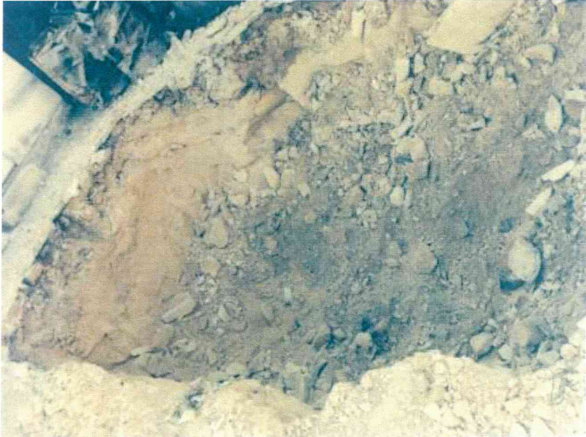
Figure 9: View of the other excavated area for the 2nd oil interceptor
