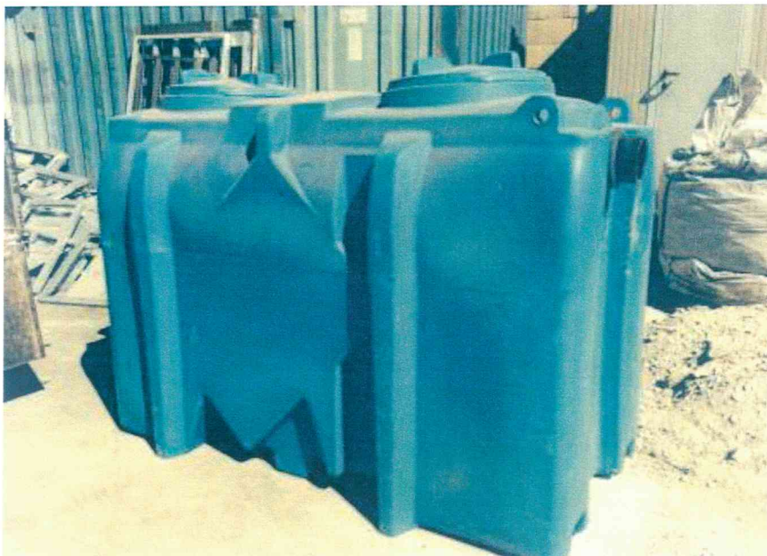
Figure 8: View of the oil interceptor prior to installation
