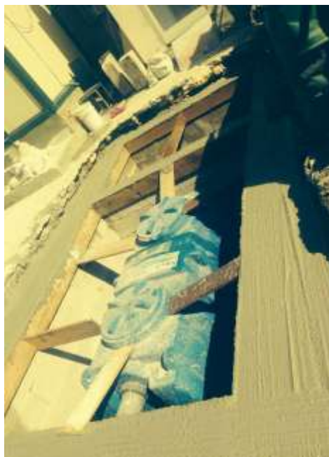
Figure 5: View of one of the installed oil separators during the back filling process
