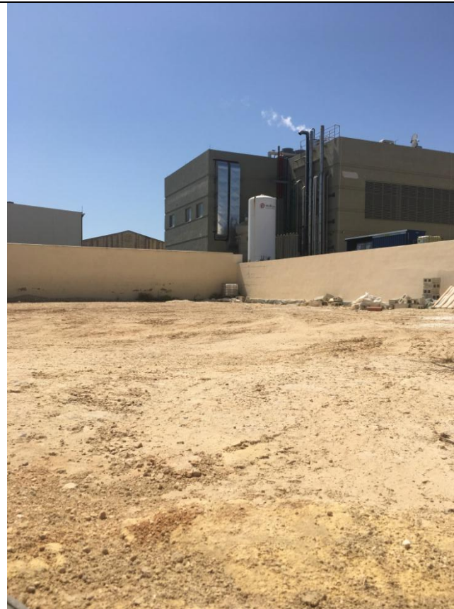
Existing site to the northwest of Sterling Chemical main building (HF50)
