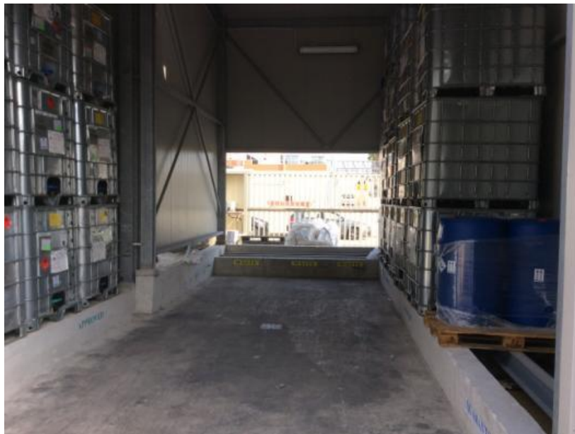
Figure 2.6: Existing external warehouse for flammable materials
