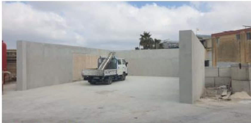
Fig 02 : View of the New enclosure
