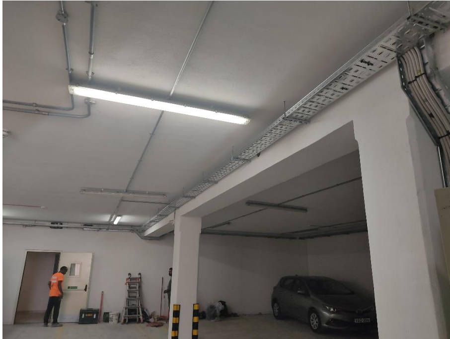
Photo 2 - Cable Containment Installation
