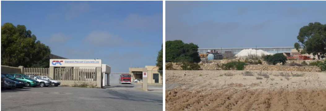
Figure 3.6: Concrete batching plants
