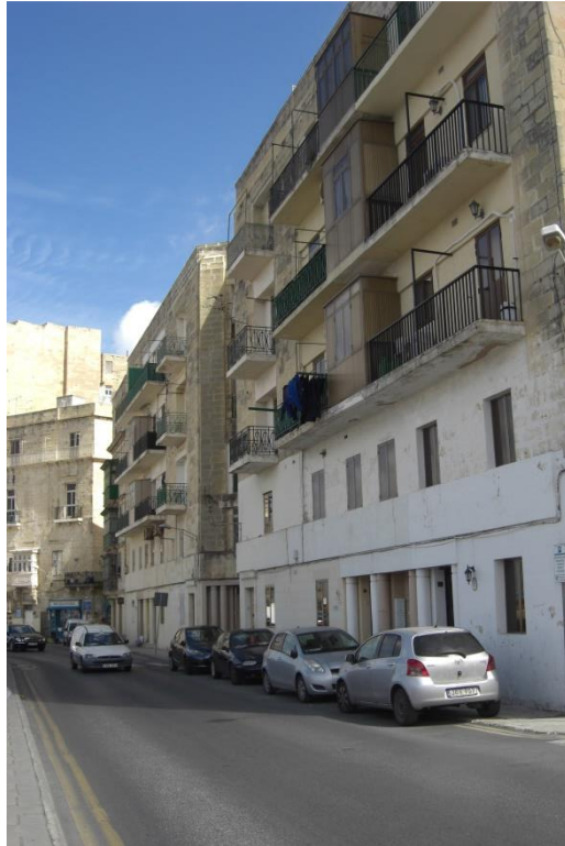
Figure 23: Apartments, Triq Marsamxett (taken on 13th March, 2018)
