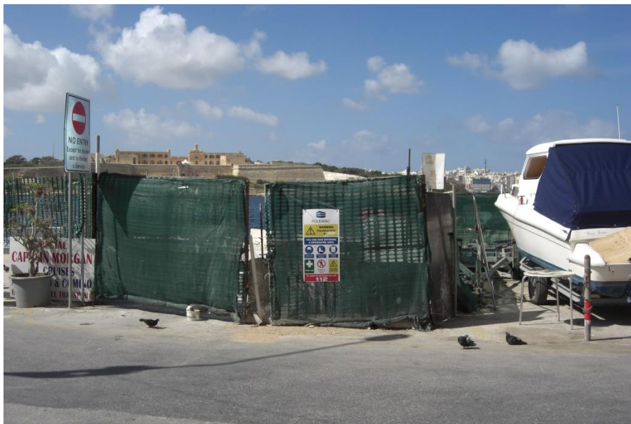
Figure 13: Construction site on the proposed scheme site (taken on 13th March, 2018)
