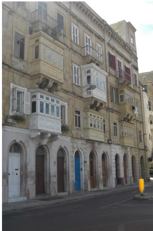
Figure 22: Traditional Maltese terraced houses, Triq Marsamxett (taken on 13th March, 2018)
