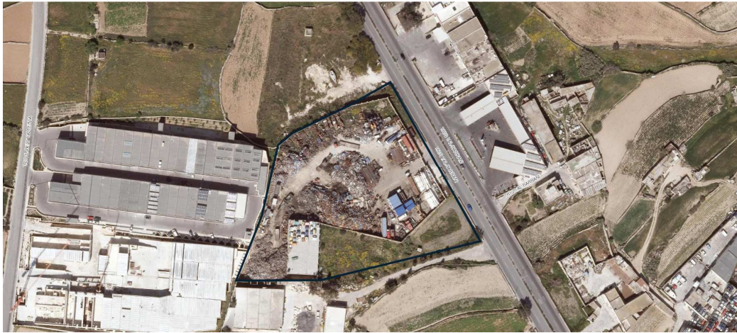
Photo 1: 2016 aerial image of entire site outlined in blue including the proposed extension. Source: PA Geoserver
