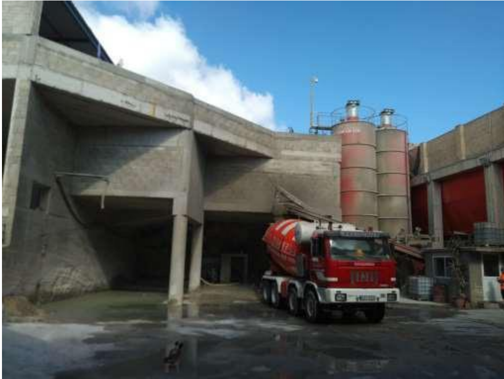
Figure03: Existing situation onsite.
