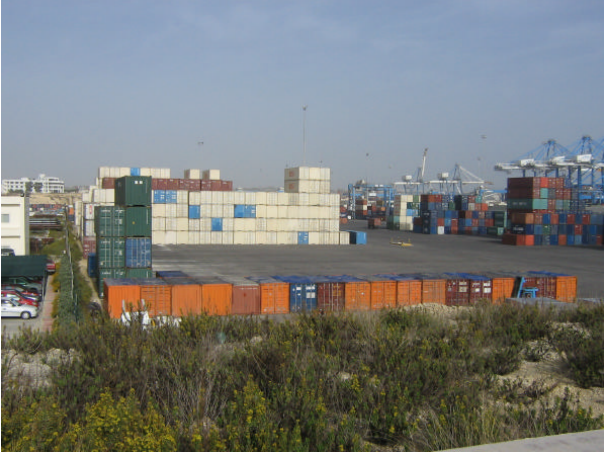
North West View
