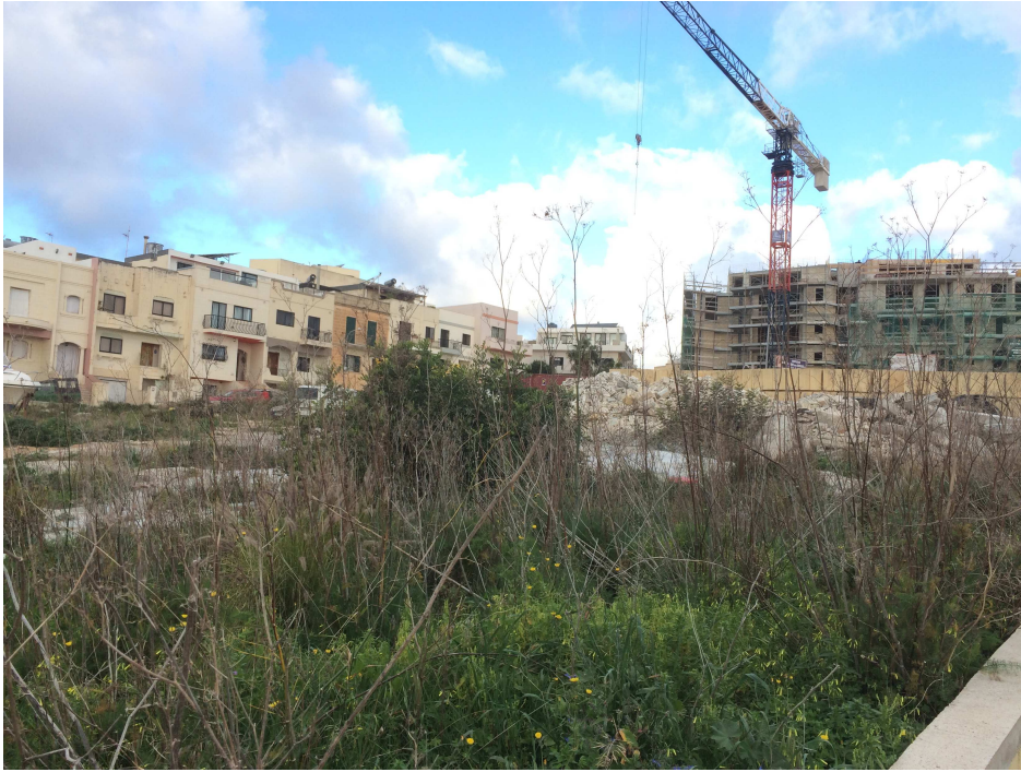
Photo 2: Site as existing Source: ERA site visit
