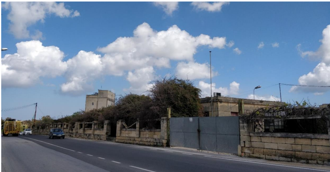
Figure 5: On-site photo taken on 28.03.2018.
