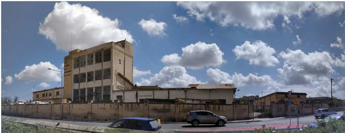
Figure 7: On-site panoramic photo taken on 28.03.2018.
