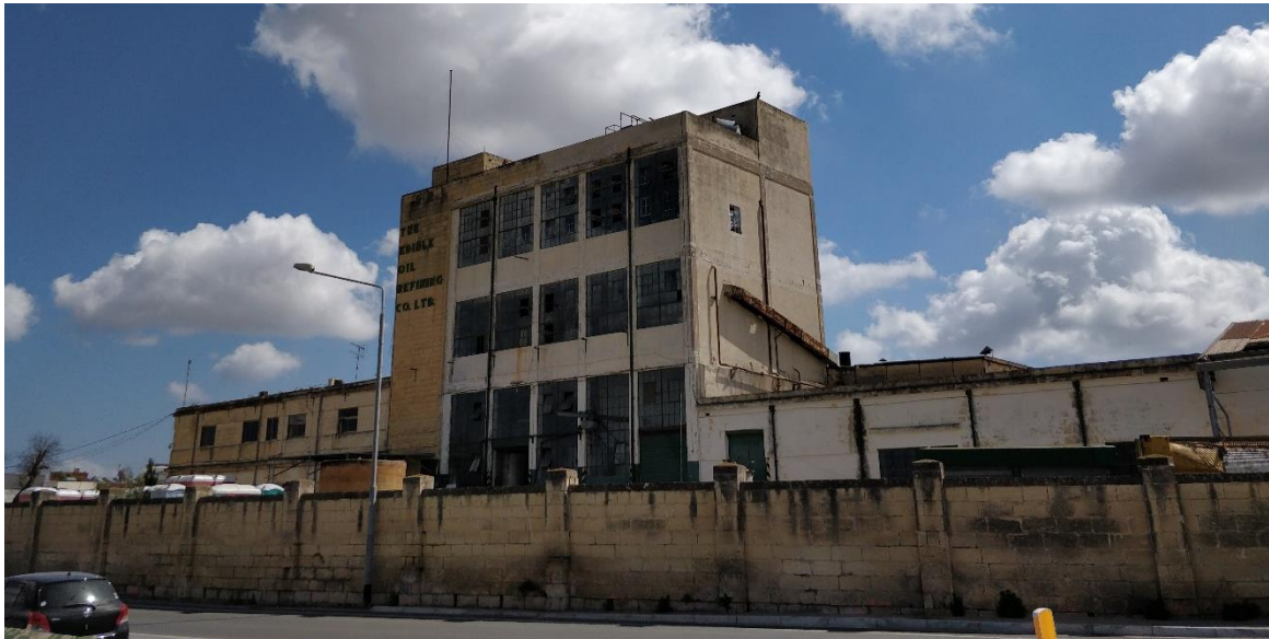
Figure 4: On-site photo taken on 28.03.2018.
