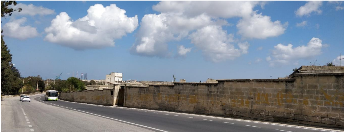
Figure 6: On-site photo taken on 28.03.2018.
