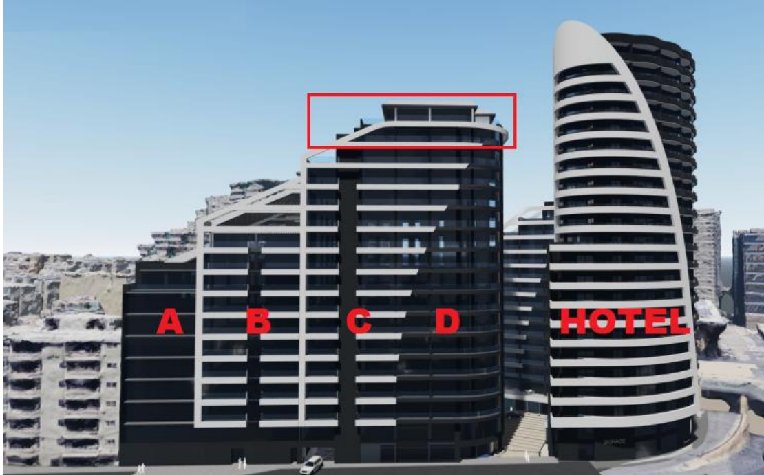
Figure 1 – Visual of proposed development with labels of block A-D and hotel tower, and proposed additional floors in red (Source: PDS. Markings in red added by ERA)
