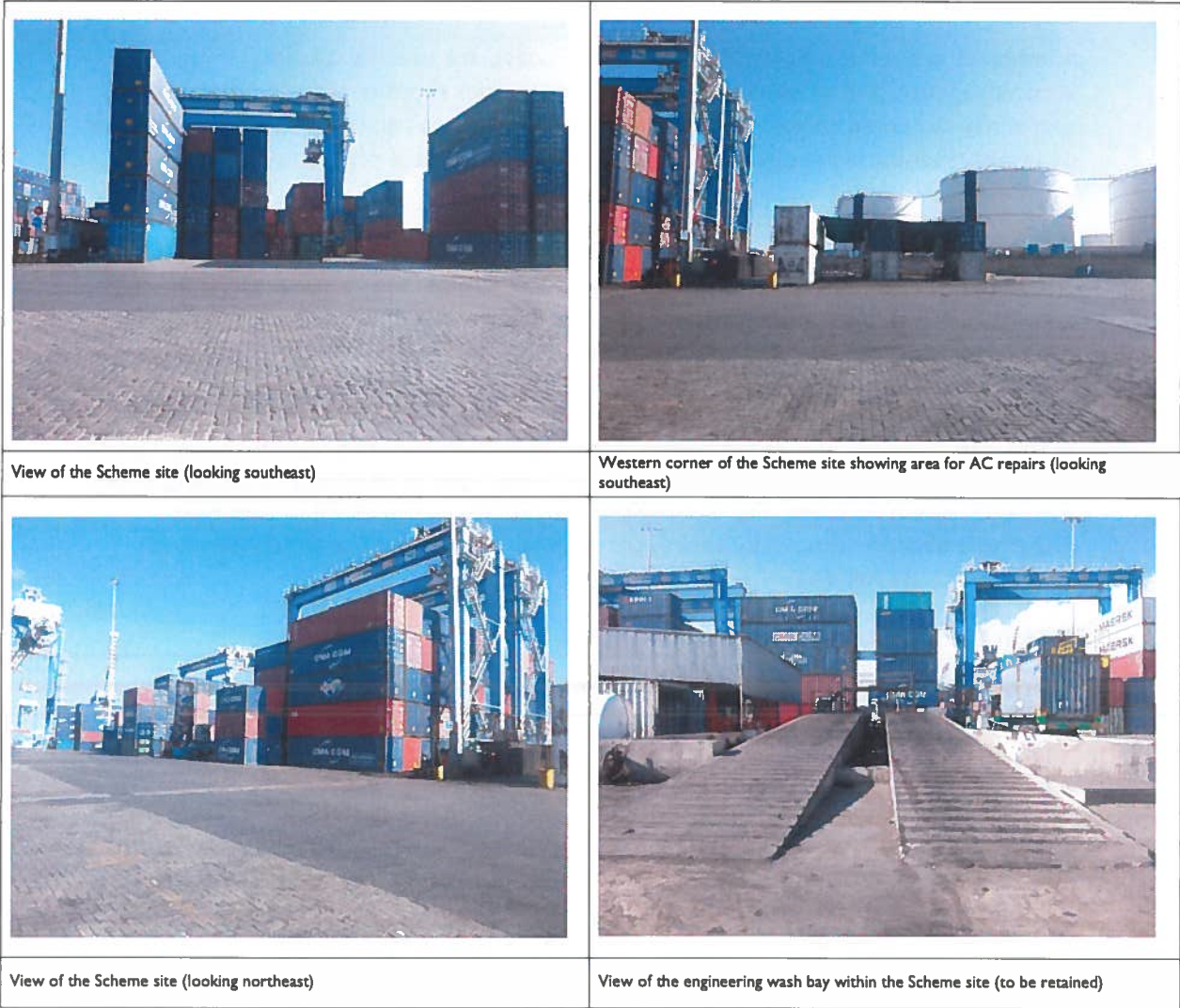
Figure 2: Images of the Scheme Site as Existing
