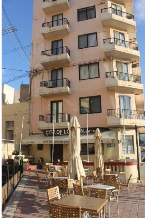
Figure 17: Bar with overlying residential units, Triq George Borg Olivier c/w Main Street (7 th January 2020)
