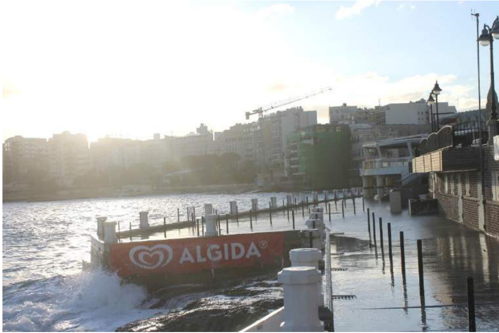
Figure 1: The San Ġiljan Aquatic Sports Club existing facilities (7th January 2020)
