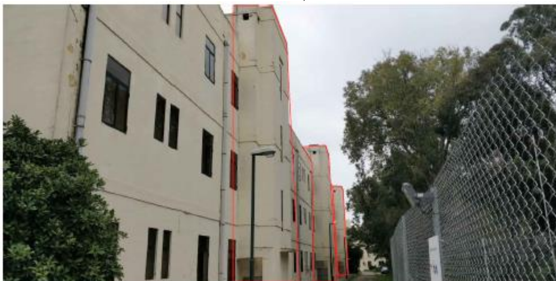
Figure 3: Photo of the rear façade showing locations of the 3 proposed lift systems marked in red (Source: E-apps PA/06875/19/45f ).
