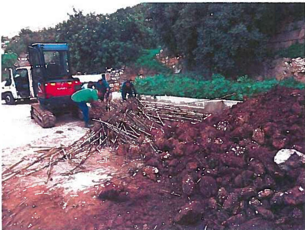
Fig. 2: Rubble stone collected from valley bed for re-use for rubble wall re-building
