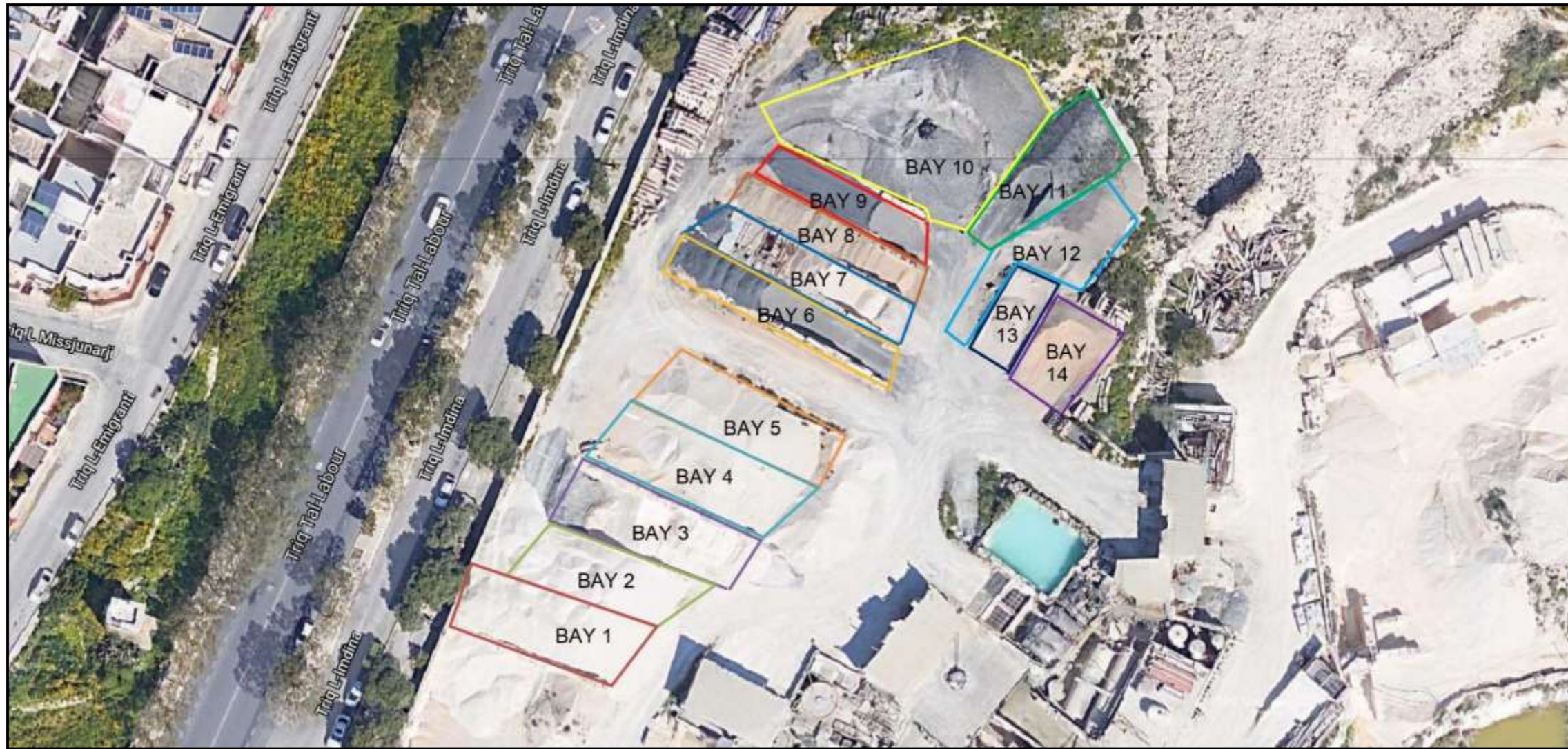
Fig. S4C: Site of installation, showing the stockpiles for plant production for the carrying out of the activities specified in Condition 1.1.1. The extent of the site boundary is indicative and shall not be used for interpretation purposes. The height of the stockpiles is to be kept below the boundary wall.
