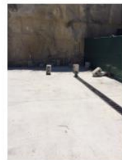
1. HPU Area- hard standing with catchment drain and pit
