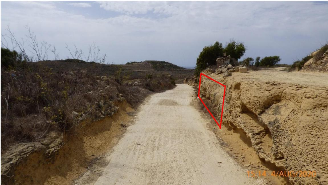
*Figure 17: Some rock needs to be trimmed to widen the road (2.4 square metres).*
