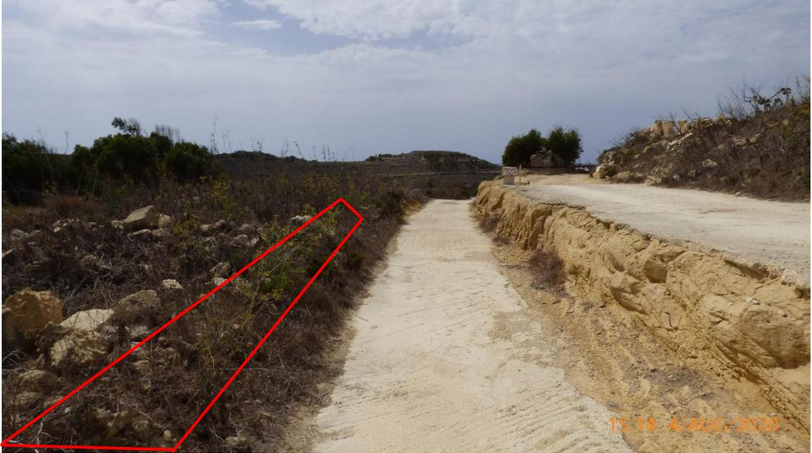
*Figure 15: The marked rubble wall will be shifted to the field (with owner's consensus) to widen the road. Some rock trimming is also proposed.*
