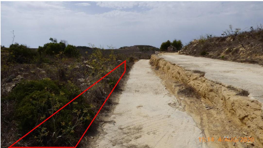
*Figure 14: The area indicated need to be widened. Part of the existing rubble need to be rebuilt. Trimming of rock is also required to lower the rock to the existing road level.*
