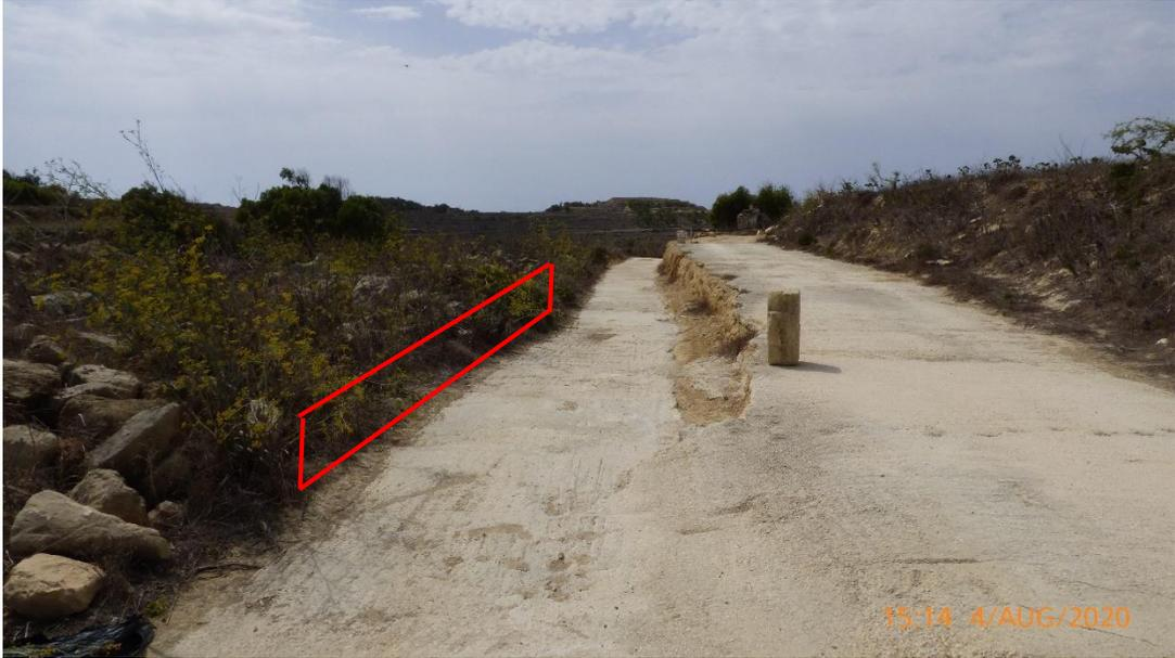
*Figure 13: Widening the road and building against the rubble wall.*
