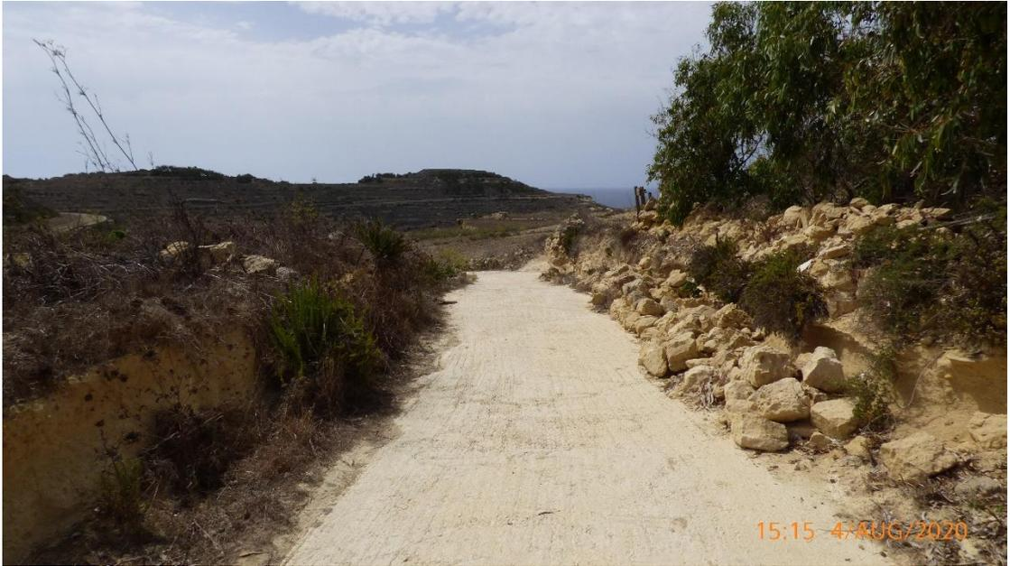
*Figure 18: Third party dilapidated rubble walls to be restored.*
