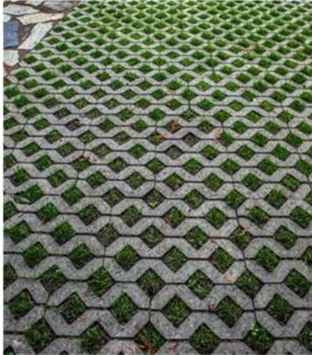
Figure 3: Mixed concrete paving and grass to enhance permeability aiding in rainwater storage.
