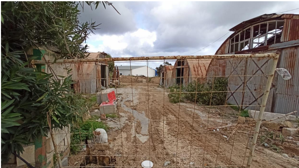
Figure 7: Photo taken during a site visit showing the Nissen huts (December 2020)
