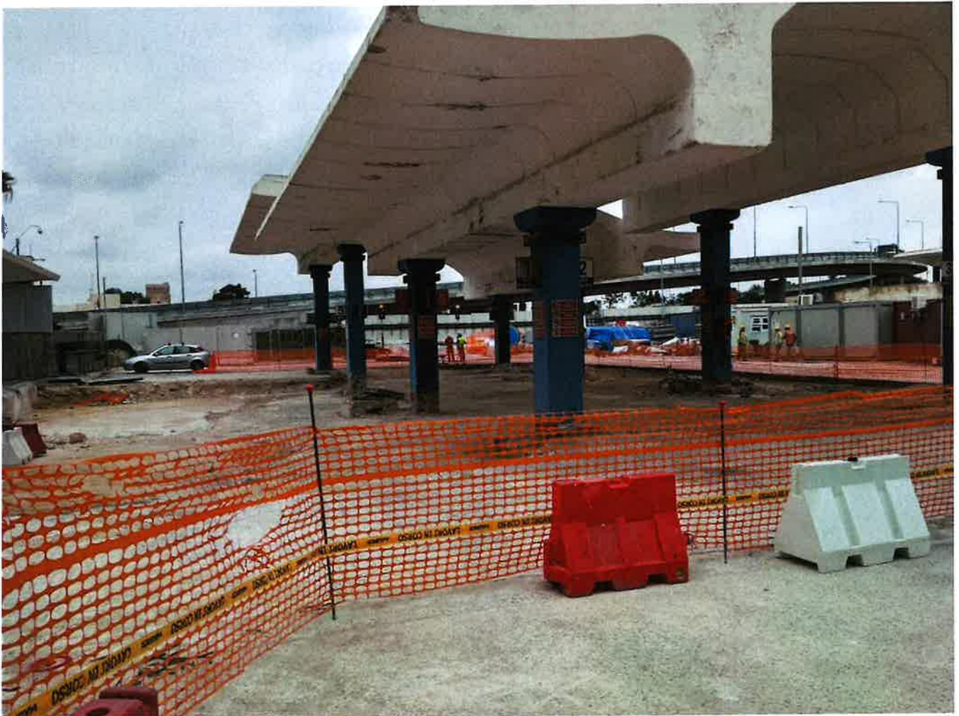
Figure 5: Photograph showing the present conditions at the Service Station
