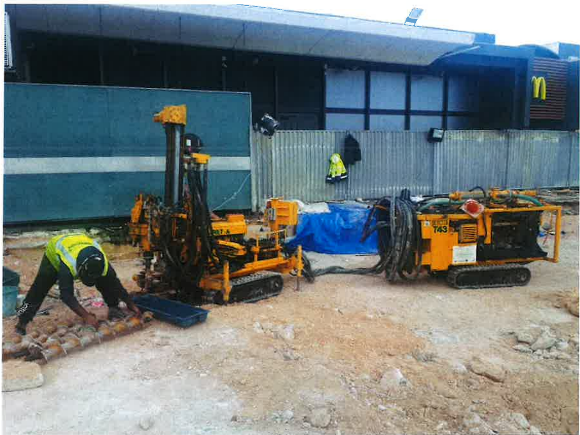
Figure 19: Beretta T43 drill rig fitted with an auger for dry drilling
