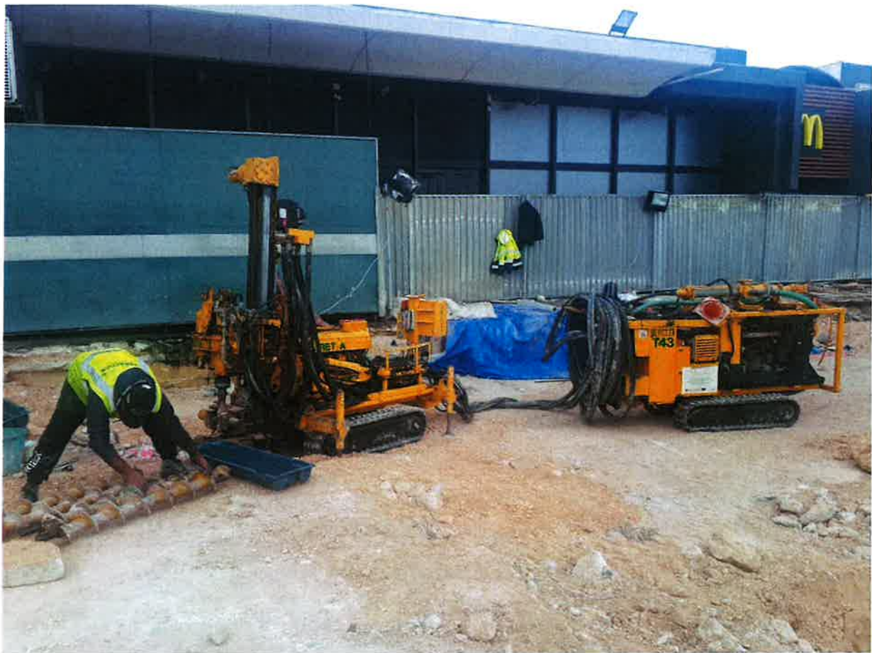
Figure 2: Beretta T43 drill rig fitted with an auger for dry drilling
