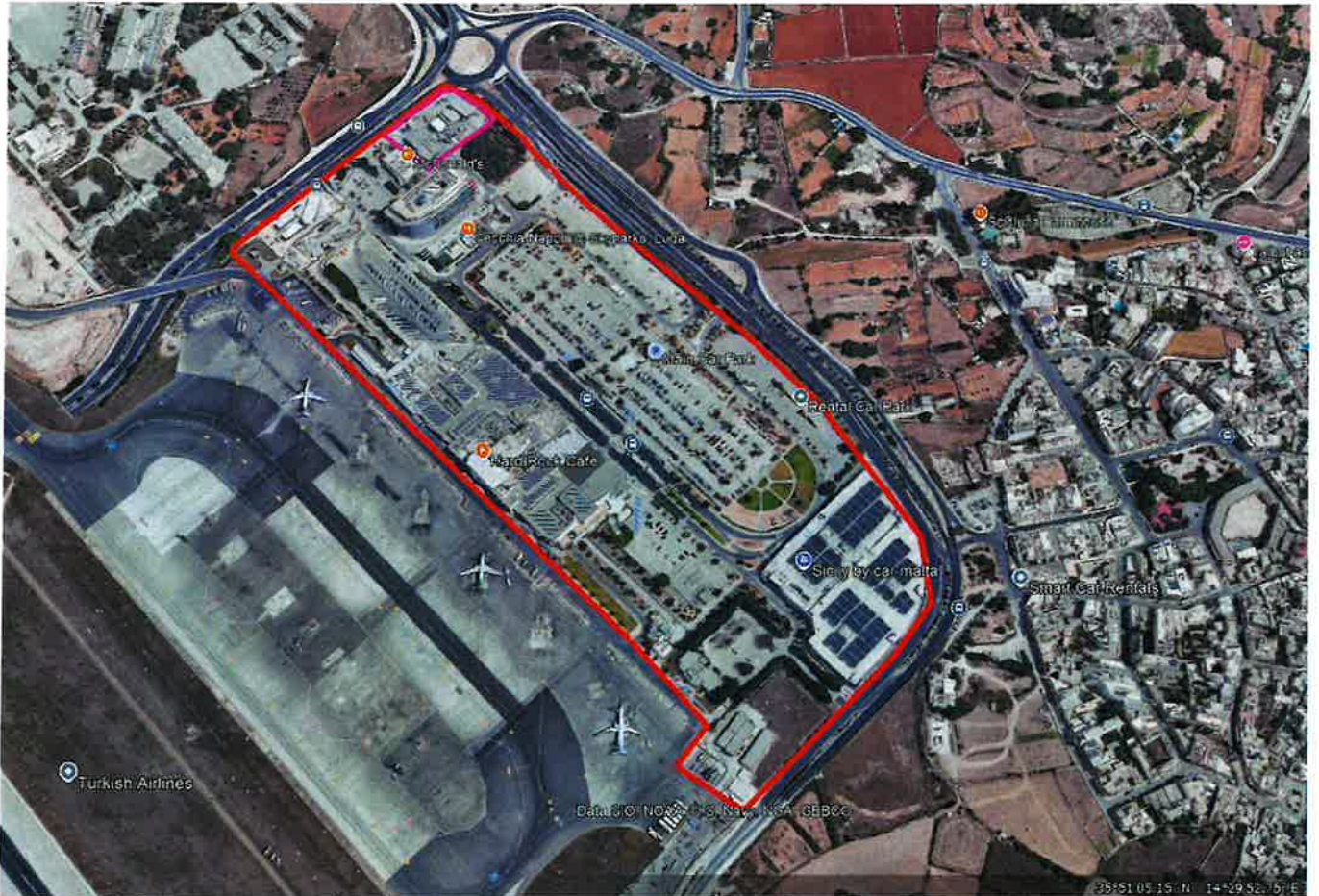
Figure 1: Google Image showing the Skyparks 2 Site. The Purple line shows the location of the Service Station
