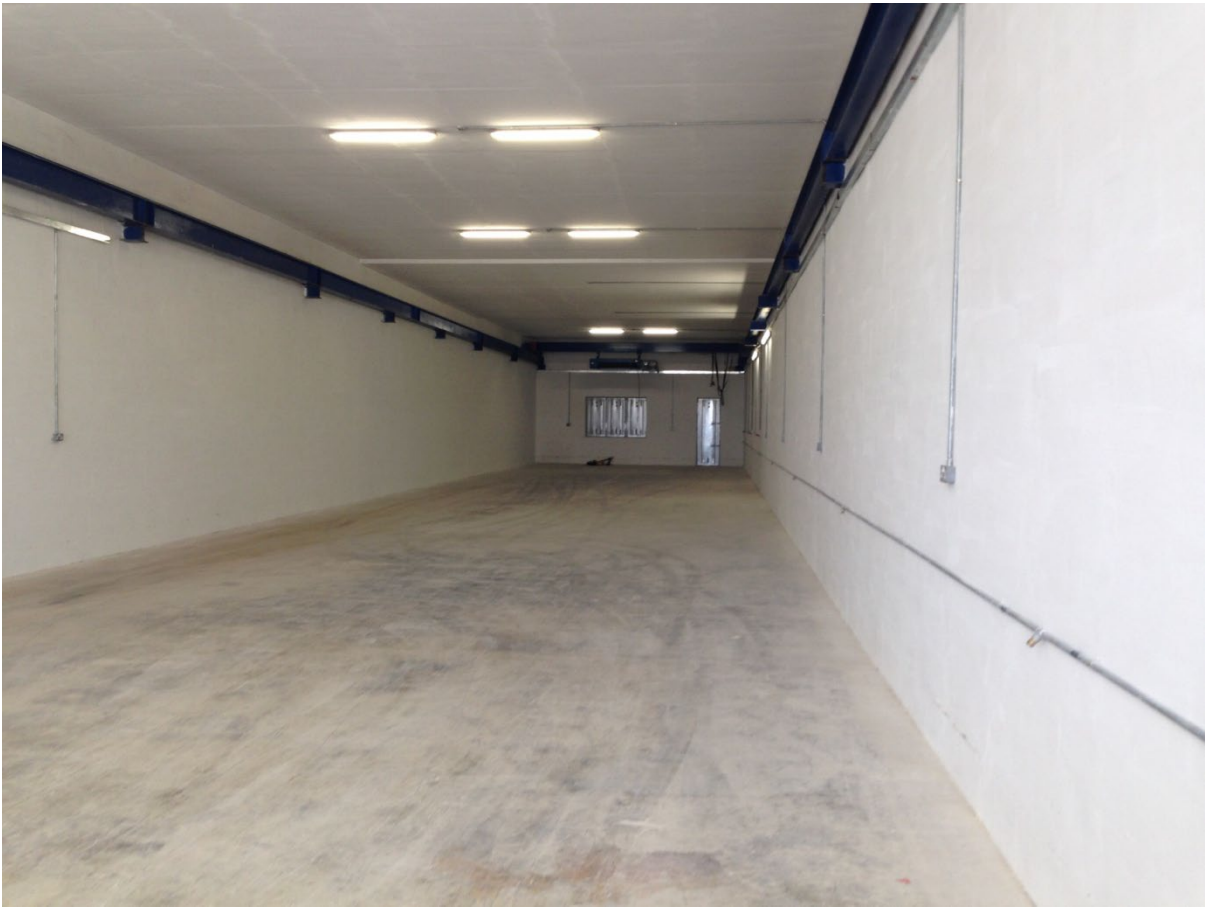
Interior of Unit
