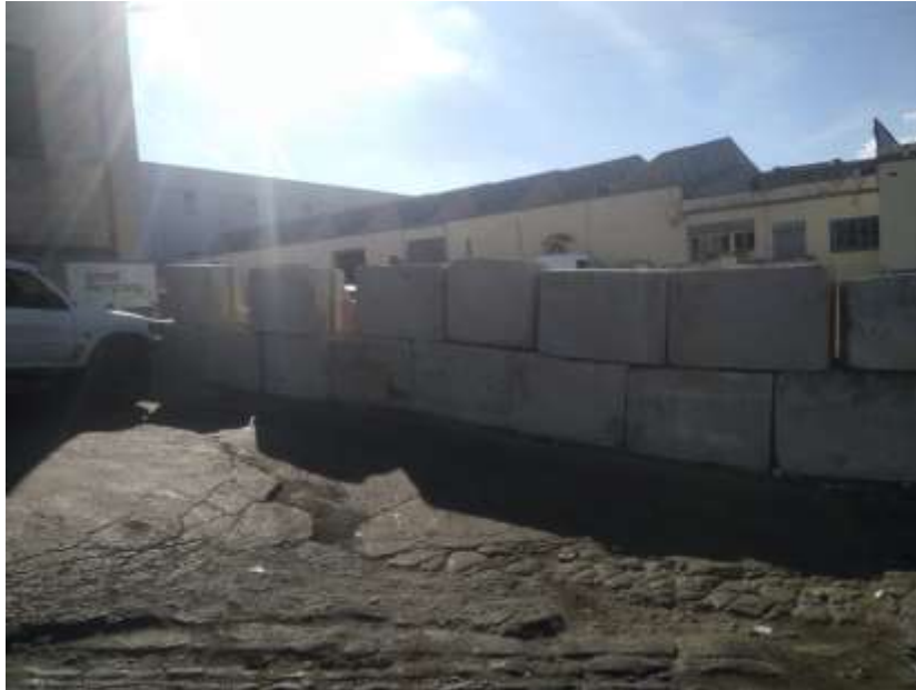
Image 16 – blocked access to the front of the site
