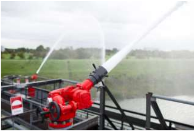
Image 3 – example of fixed fire monitor
