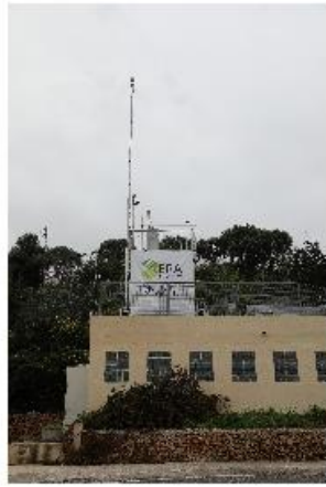
St Paul's Bay Station
