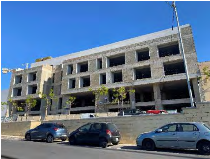
Developments under construction
