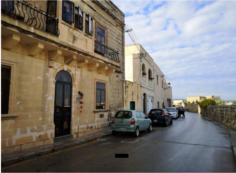
FIGURE 11: RESIDENTIAL PROPERTIES LOCATED RELATIVELY CLOSE TO QUARRY TAS-SEJBA (DECEMBER 2020)
