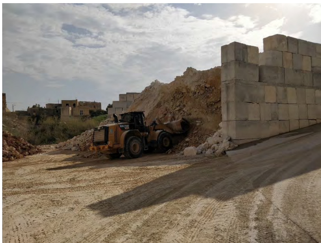
FIGURE 22: MATERIAL STOCKPILES (AUGUST 2020)
