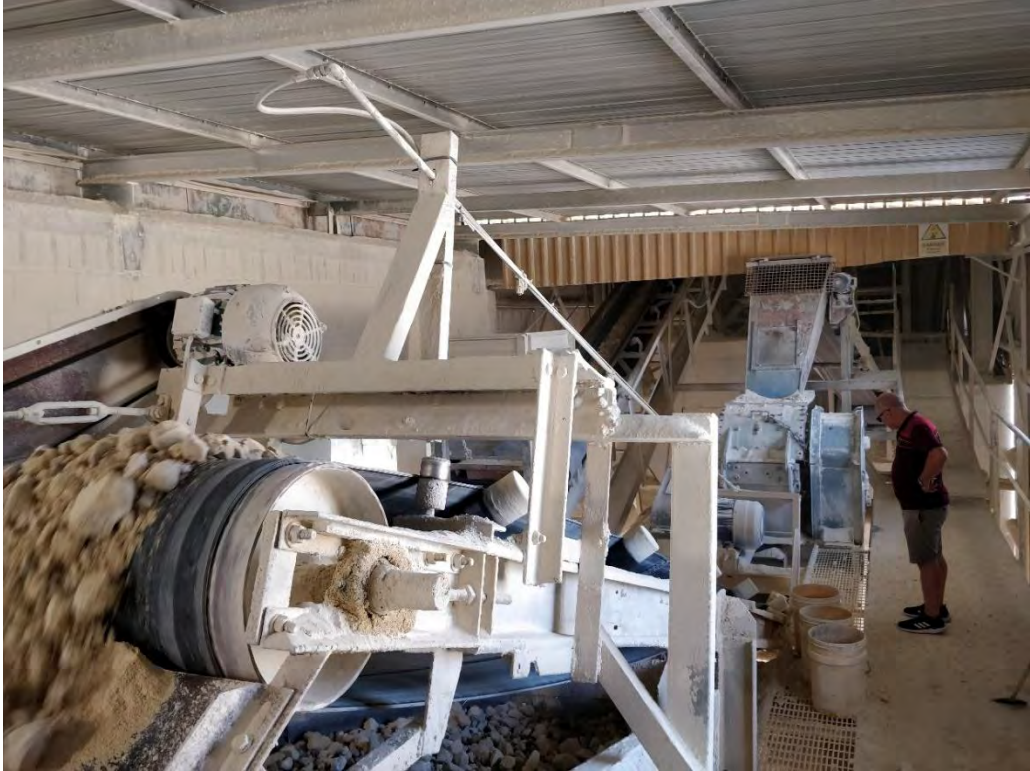
FIGURE 21: MATERIAL CRUSHING OPERATIONS (AUGUST 2020)
