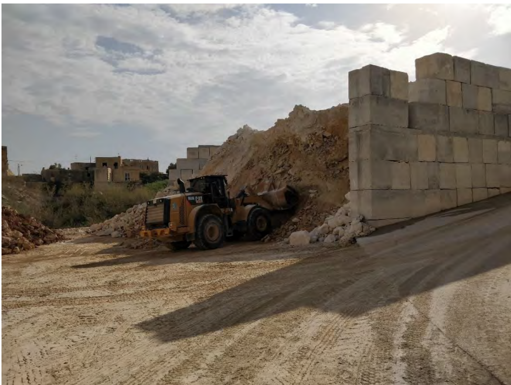
FIGURE 22: MATERIAL STOCKPILES (AUGUST 2020)
