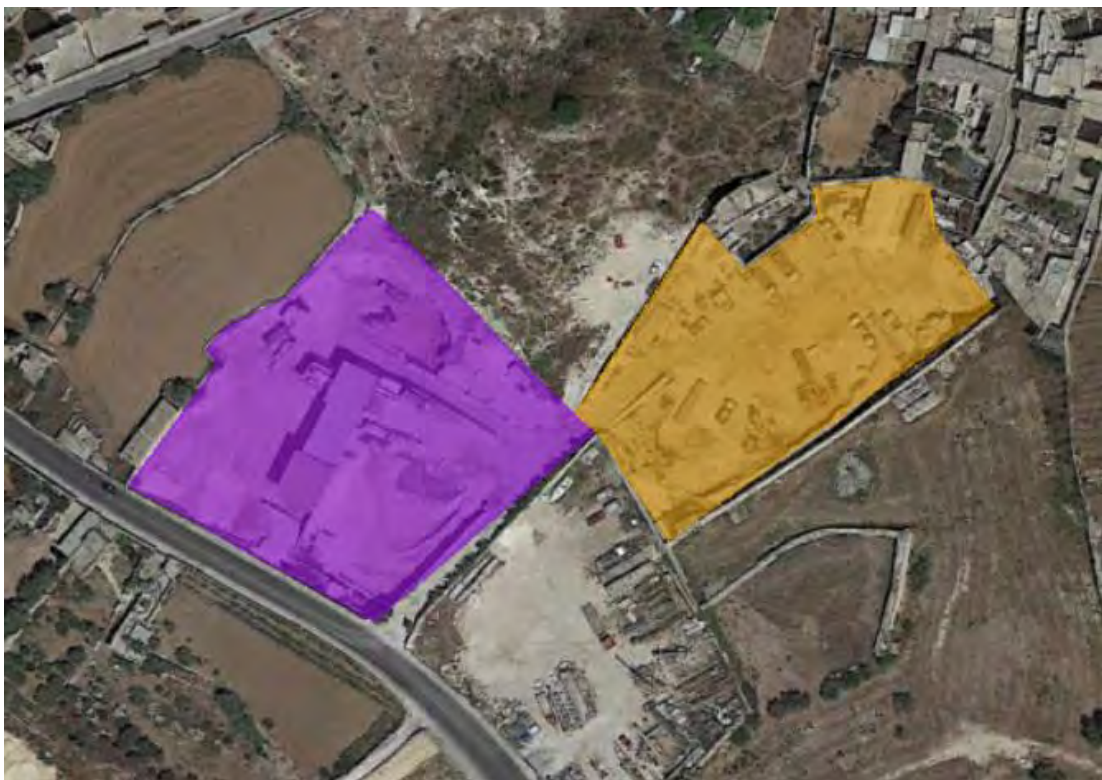
FIGURE 3: DIVISION OF SITE FOR EASE OF REPORT. EAST: ORANGE AND WEST: PURPLE
