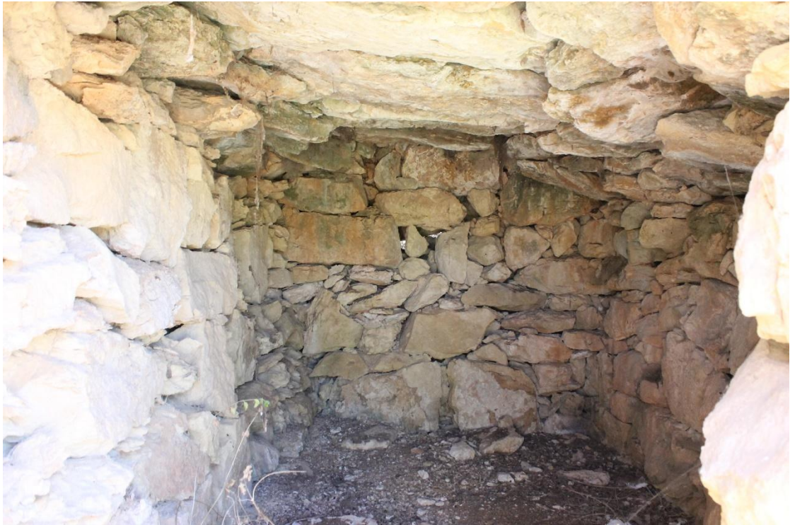
Figure 32: Feature B, Intern of corbelled stone hut (Girna)
