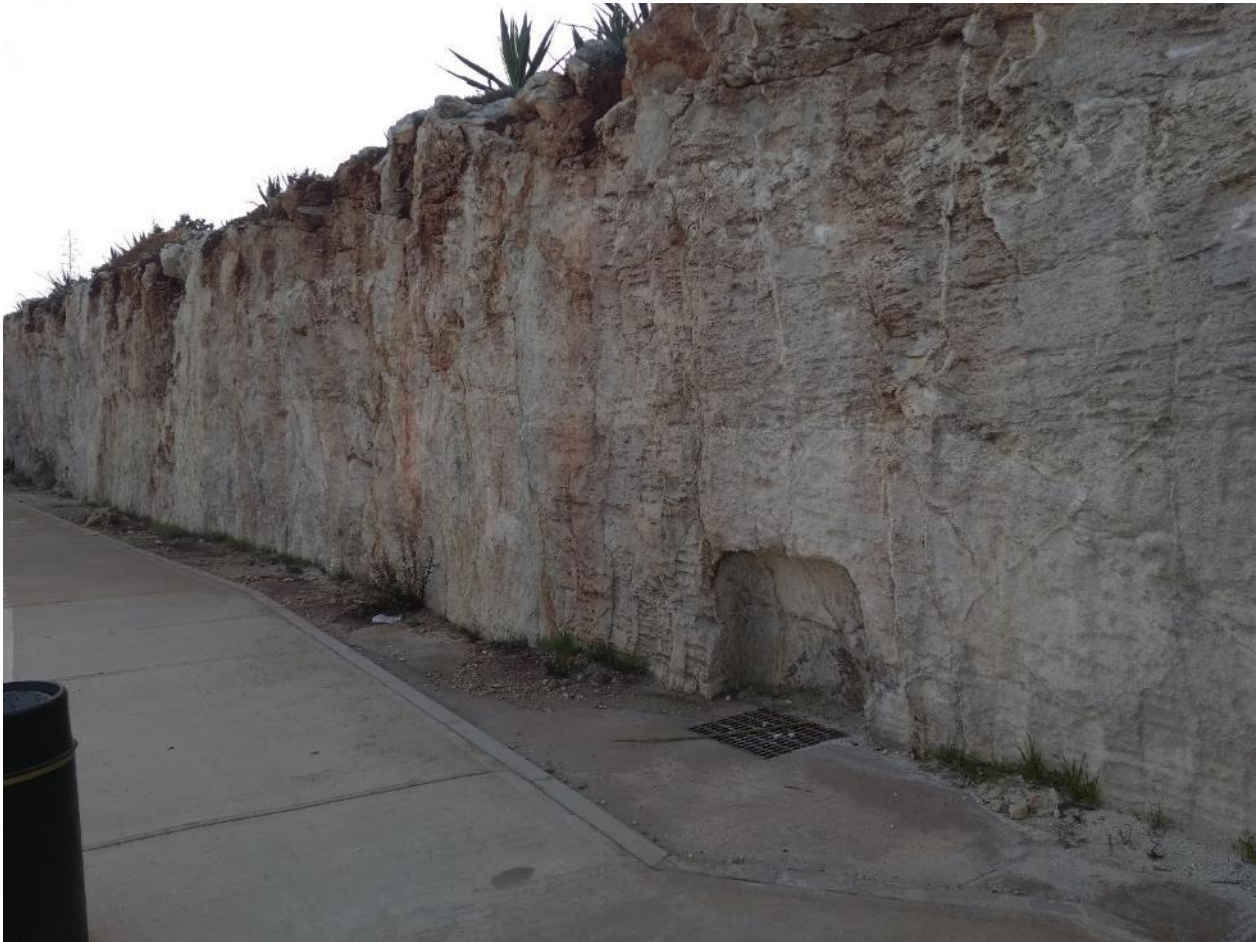
Figure 15: Coast Road cutting about 4m high exposing strata of the Xlendi Mb (Note the typical cross bedding)
