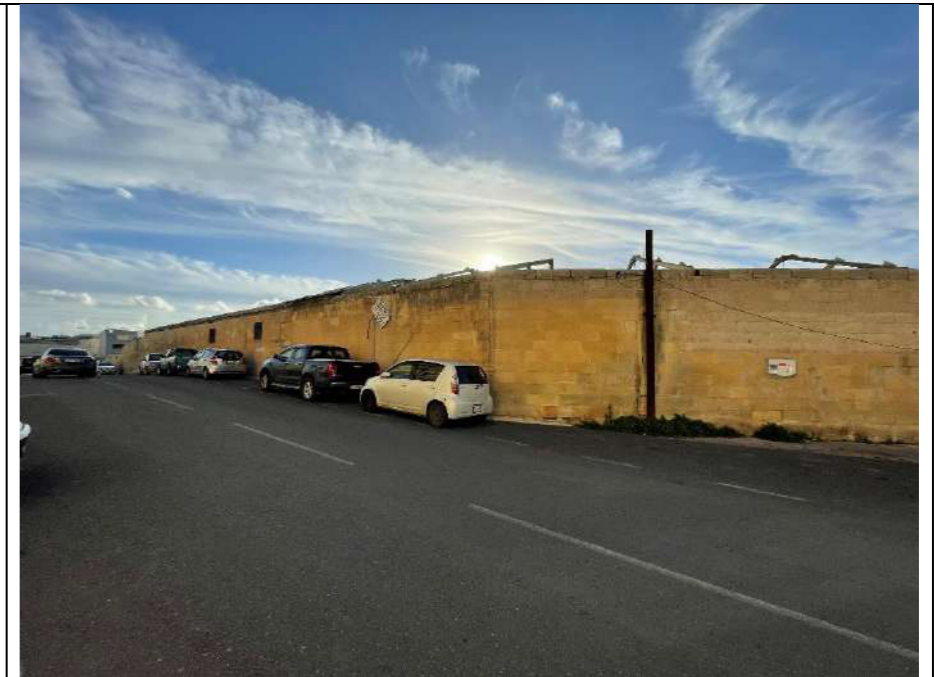
Northeast corner of the Scheme site (looking south)
