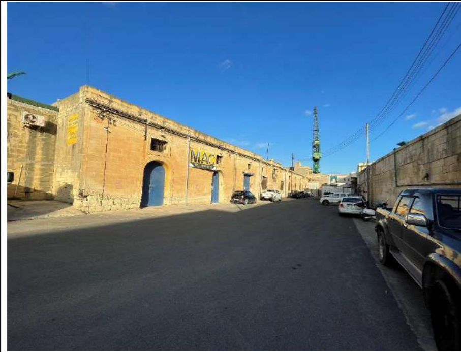
Older warehousing development on Triq Garrick
