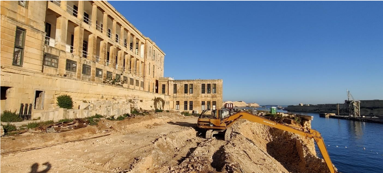
Images showing the fill material proposed to be removed and excavated.
