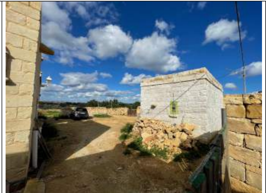
Smaller building (looking north from the entrance to the Scheme site)
