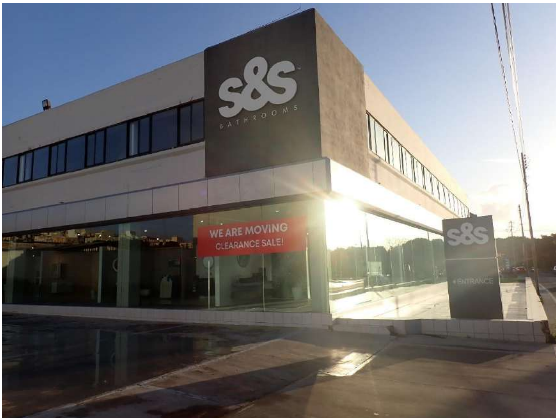
FIGURE 4: EXISTING S&S SHOWROOM, TRIQ IL-MOSTA (4 TH DECEMBER 2024)
