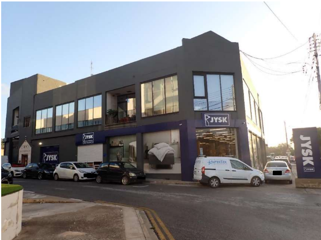
FIGURE 12: NEIGHBOURING COMMERCIAL OUTLET WITH OVERLYING OFFICES (4 TH DECEMBER 2024)
