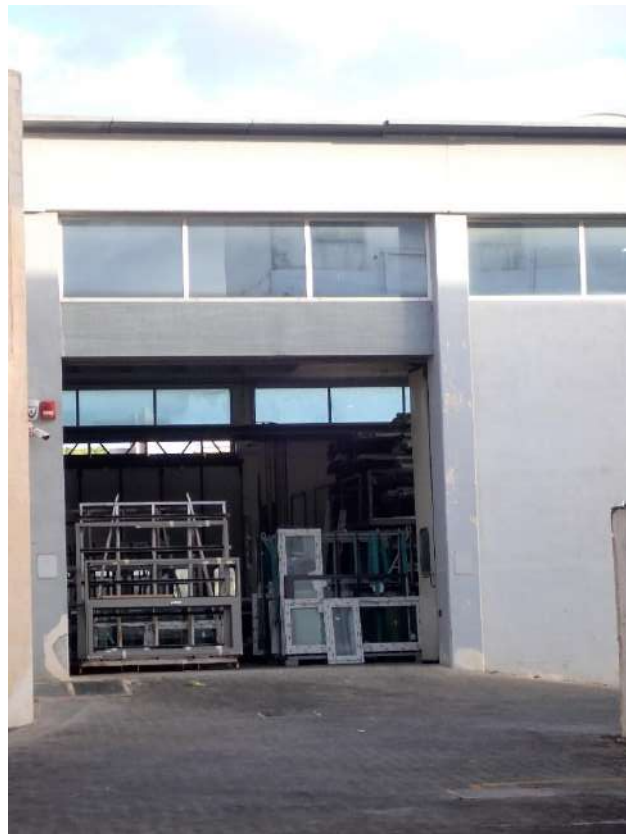
FIGURE 16: SMALL INDUSTRIAL WAREHOUSE/WORKSHOP
