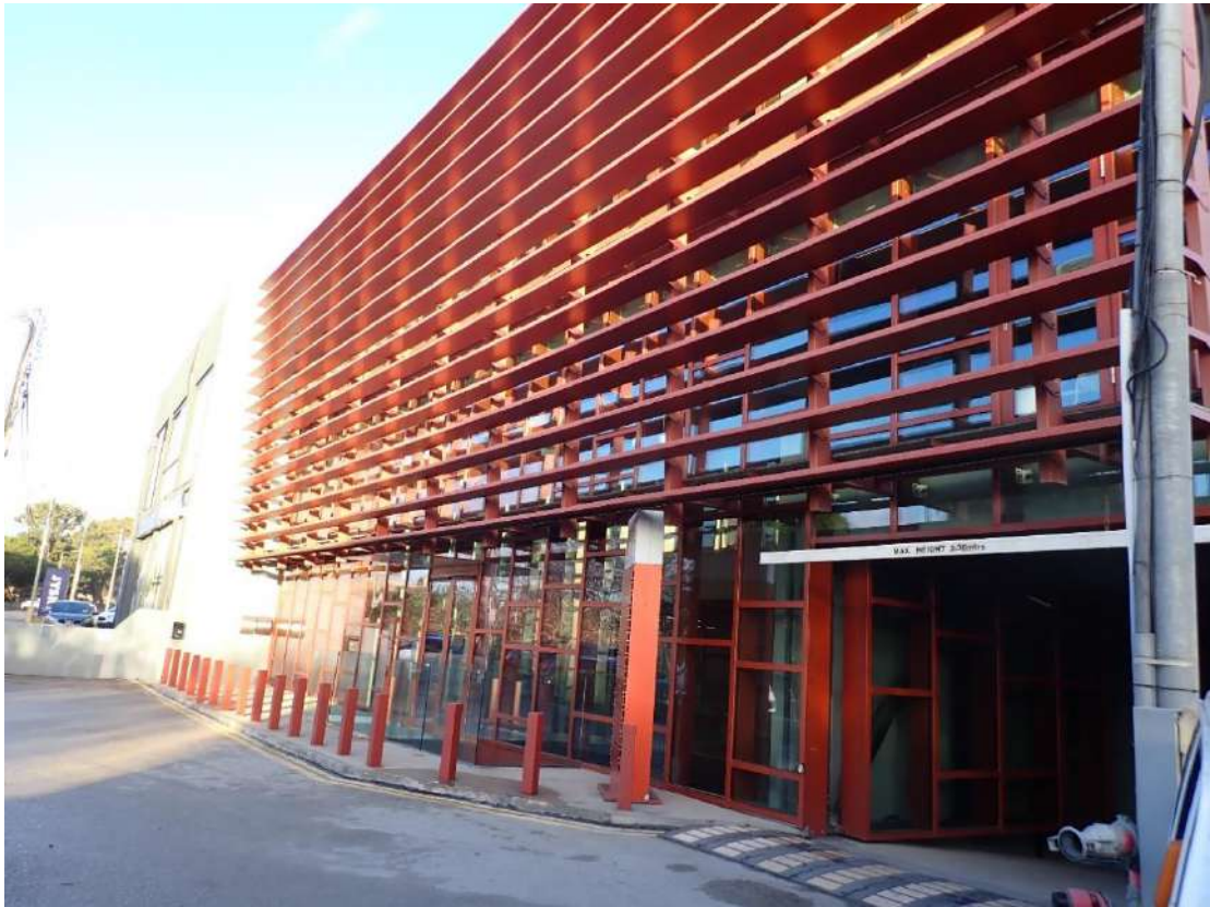
FIGURE 15: OFFICE BLOCK BUILDING (4 TH DECEMBER 2024)
