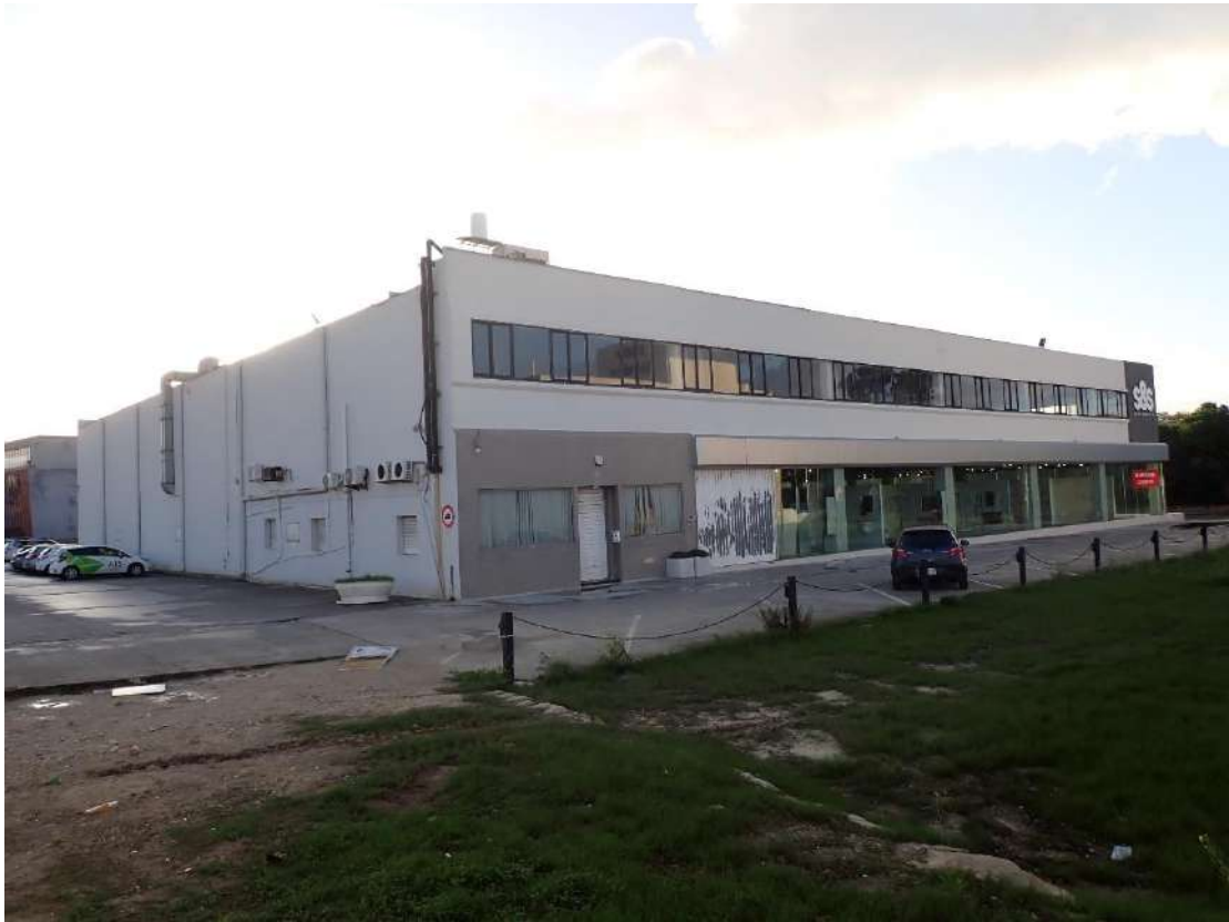
FIGURE 11: EXISTING S&S SHOWROOM, PARKING AND OPEN AREAS (4 TH DECEMBER 2024)
