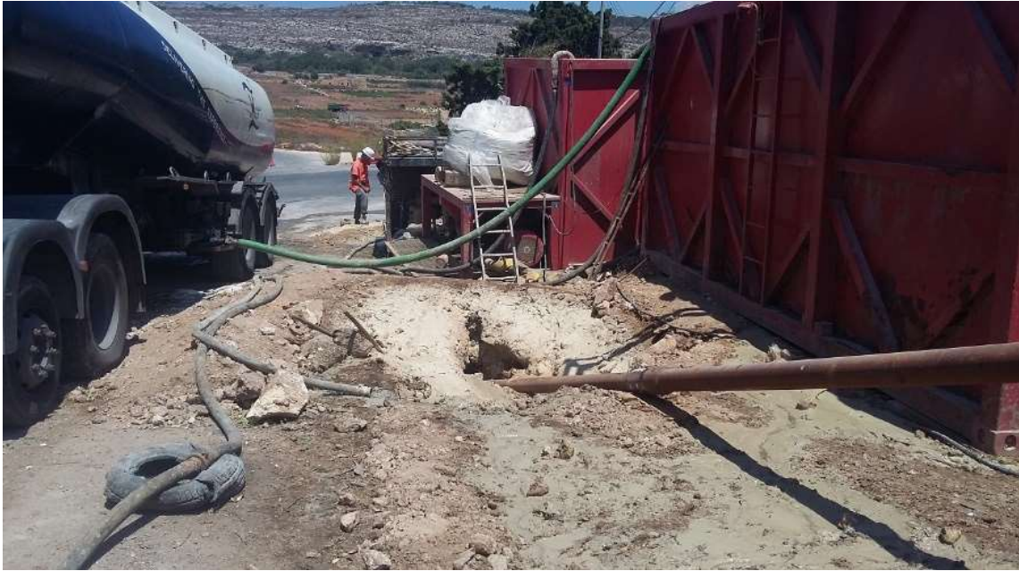
materials and equipment on each node
