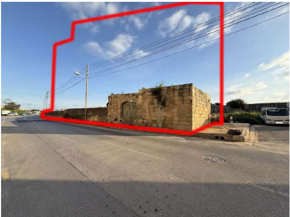
FIGURE 7: BUILDING AT THE NORTHWEST CORNER OF THE PLOT
