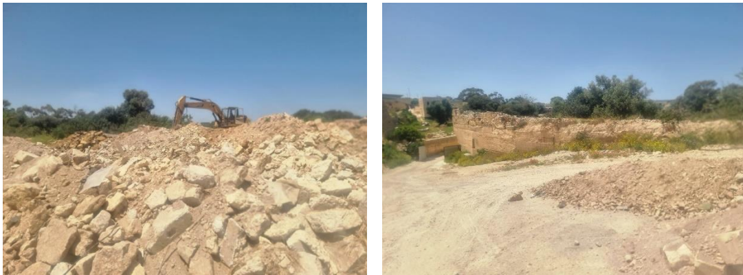
FIGURE 9: CURRENT CONDITION OF THE SCHEME SITE
